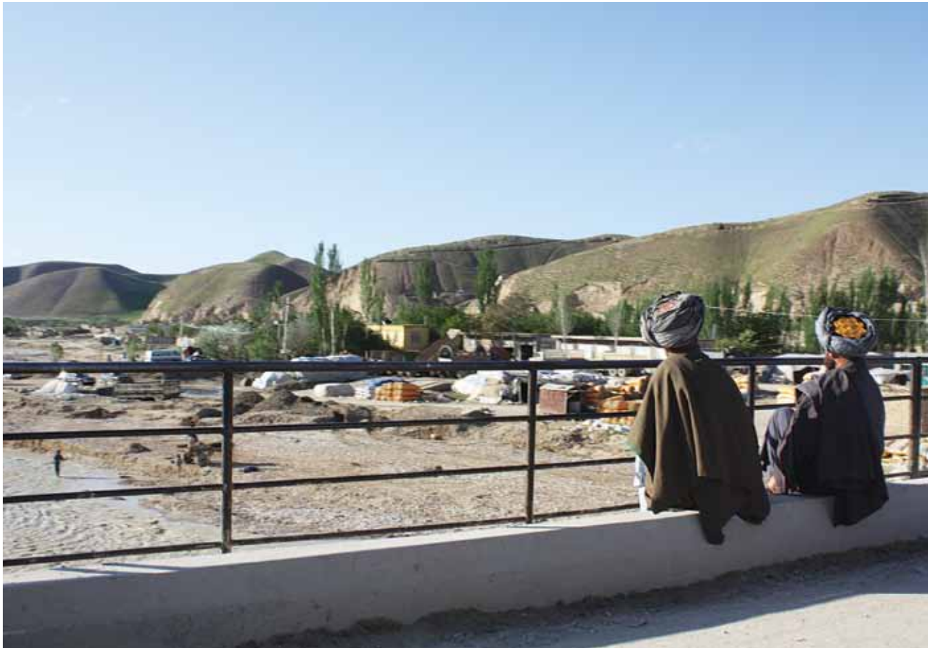
The bridge over the Maimana River
