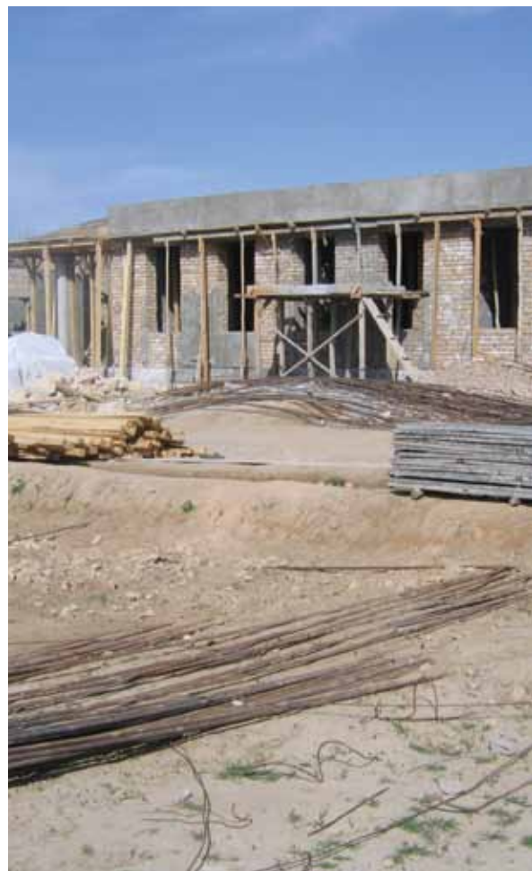
School construction in Khwoja Namusa, Pashtun Kot
