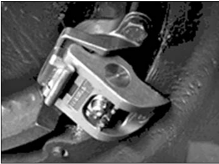
FIGURE 15-1A In the locked position from inside the manhole.
