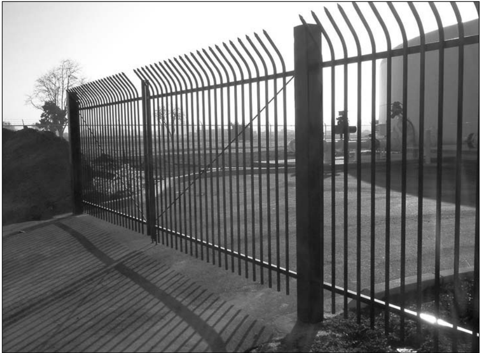
FIGURE 3-4 Wrought-iron perimeter fence
