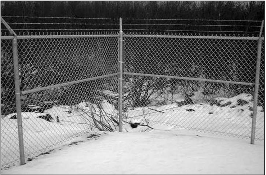
FIGURE 3-1 Security fence corner with truss braces & tension rods
