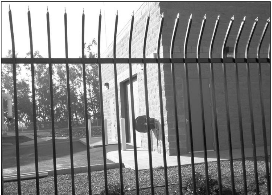
FIGURE 3-3 Example of a wrought-iron fence
